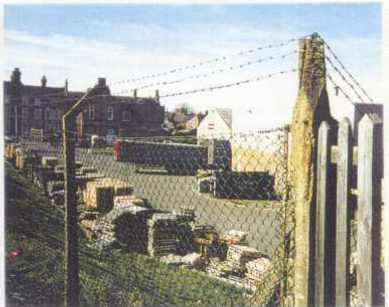
developing new facilities on the 3M site
