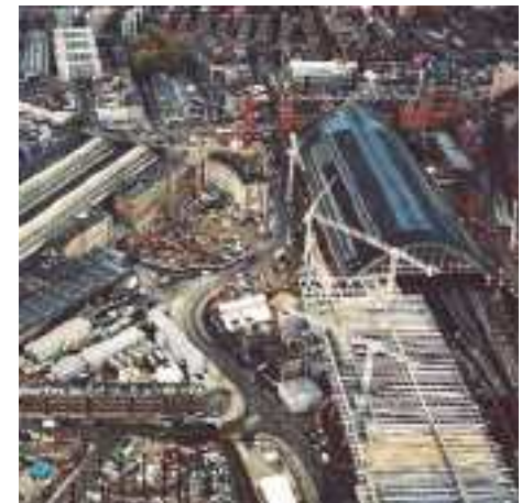
fig.119 St Pancras International Station under construction.
