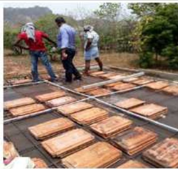
Placement of clay tile
