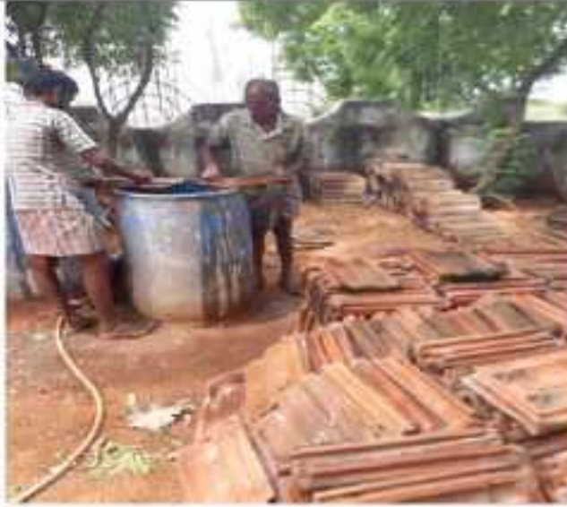
Washing of Clay tile before use
