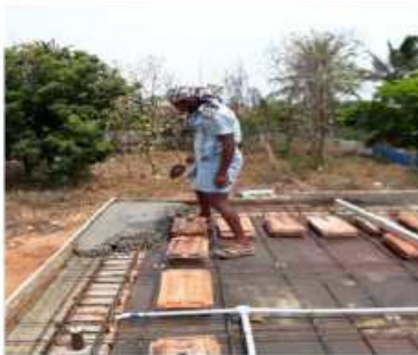
Filled with RCC layer
