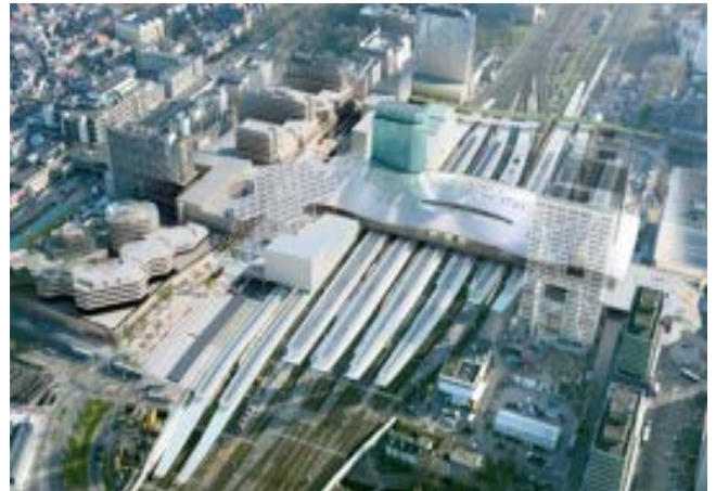
Utrecht Central Station
