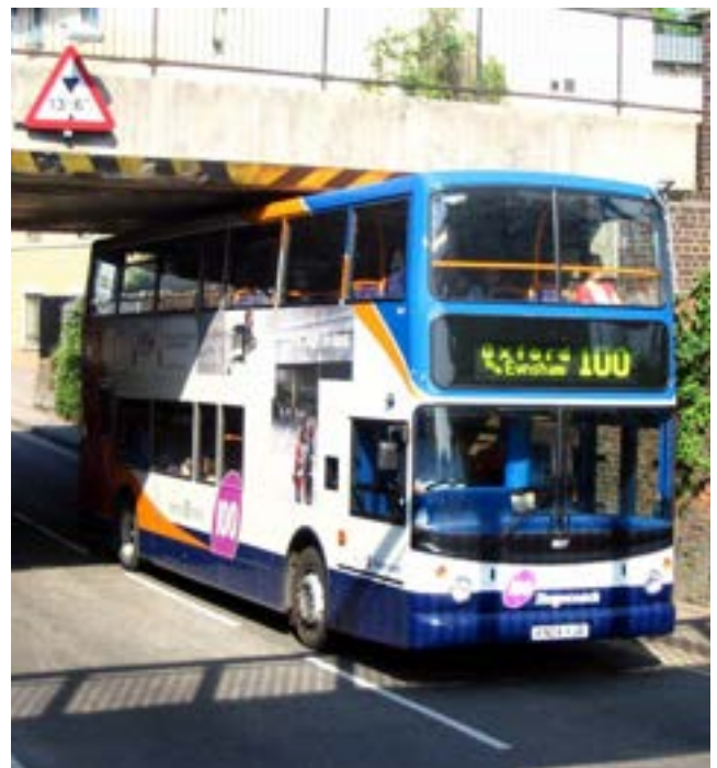
Tight fit under Botley Road Bridge
