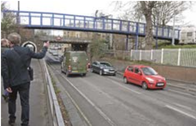
Pedestrian path over Botley Road
