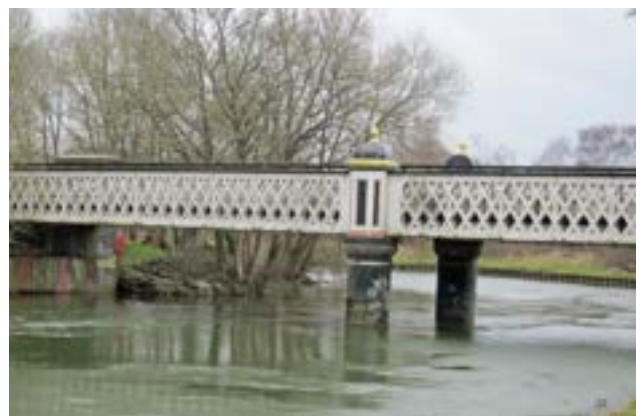
Gas works Bridge
